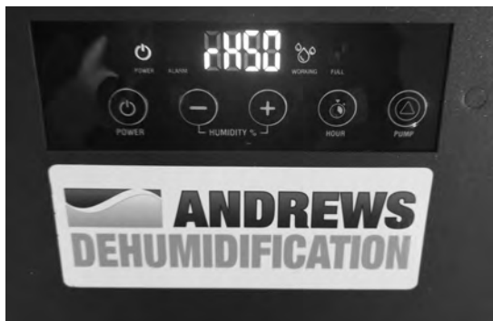
Fig 3 : Switch on the unit via the front panel and set the desired humidity via the up and down arrows
