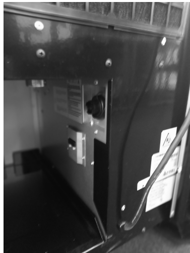
Fig 5 : The condensate pump is close coupled electrically to the machine via a built in auxiliary connection. Remove the internal tank at the back of the unit and then the power plug can be seen. On the front control panel you must push the button that says pump. This will avoid the unit from stopping when you remove the internal tank.
